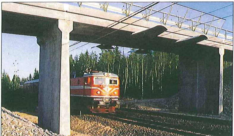
Skanska Prefab's new bridge-building system enables the National Rail Administration to replace level crossings with overpasses while minimizing disruptions in train traffic. This overpass is at Malshult, between Osby and Hässleholm in southern Sweden.
